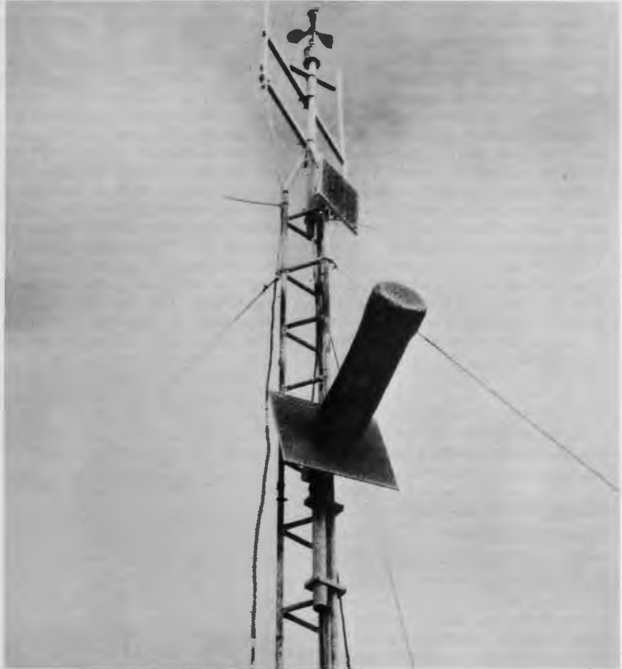
The MAPS R automatic weather station tower holds two unconventional pieces of equipment; a cylindrical antenna for broadcasting data to a geostationary satellite and, above it, a square plate holding the several circular solar energy cells which power the station.
