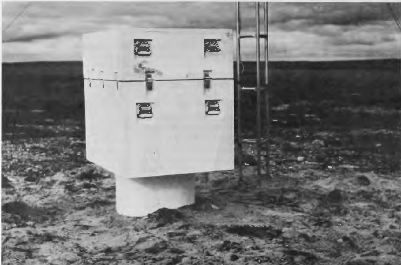
The MAPS R instrument box sits on an insulated cylindrical column containing the thermosyphon, which passively draws heat from the ground to keep the electronics at an operational temperature.
