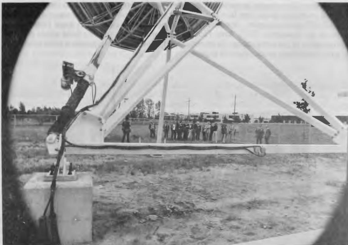
*The 10-metre dish antenna, an aid in reception of imagery from GOES-EAST geo stationary satellite, dwarfs the group of observers outside AES Downsview.*
