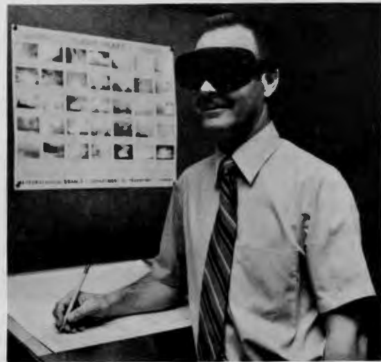
Technician L.A. MacNeill demonstrating panoramic dark adaptor goggles.
