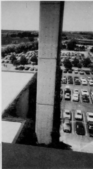
Ensnconed in the north east corner is this huge 45 metre chimney acting as the main exhaust for the boiler room. Its principal charm is the creeper plant winding its way up the side.
