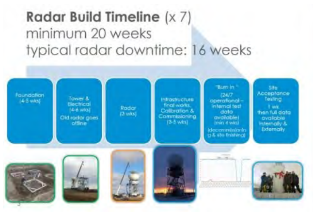
Figure 8 (left). Typical Radar Construction Timeline in 2019.
