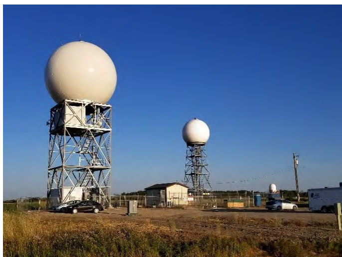
Figure 7. Foxwarren MB: Example of new S-band radar alongside old C-band radar in 2018 (with temporary X-band radar on right hand side)
