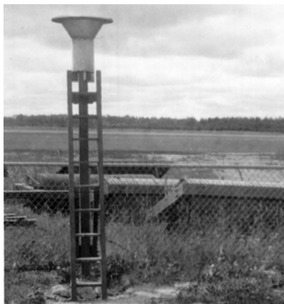
Figure 3: A similar gauge to the Brooks Shield being tested in Kapsukasing, Ont, in the 1940s.
