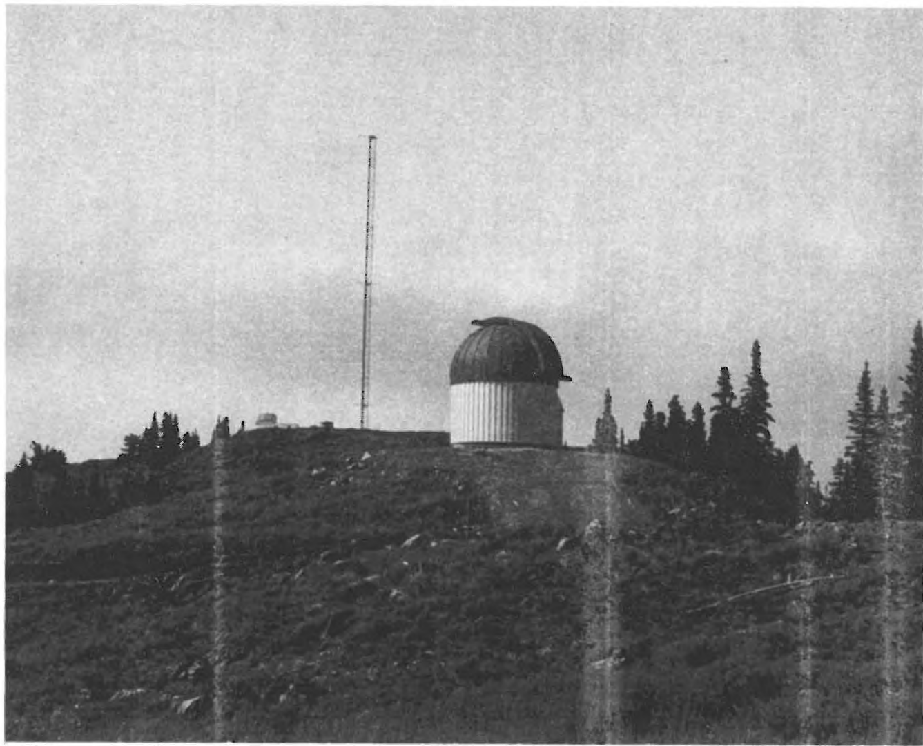
FIGURE 1. VIEW SHOWING 200 FOOT TOWER, POLARIS IMAGE MONITOR BUILDING, AND 16" TELESCOPE DOME
