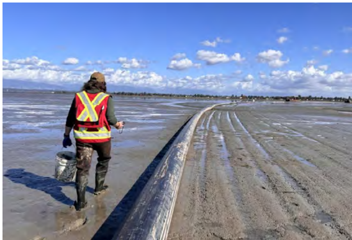
A DUC staff member walks along the temporary pipeline that brings sediment to the foreshore of the Fraser River Estuary. © Ducks Unlimited Canada
