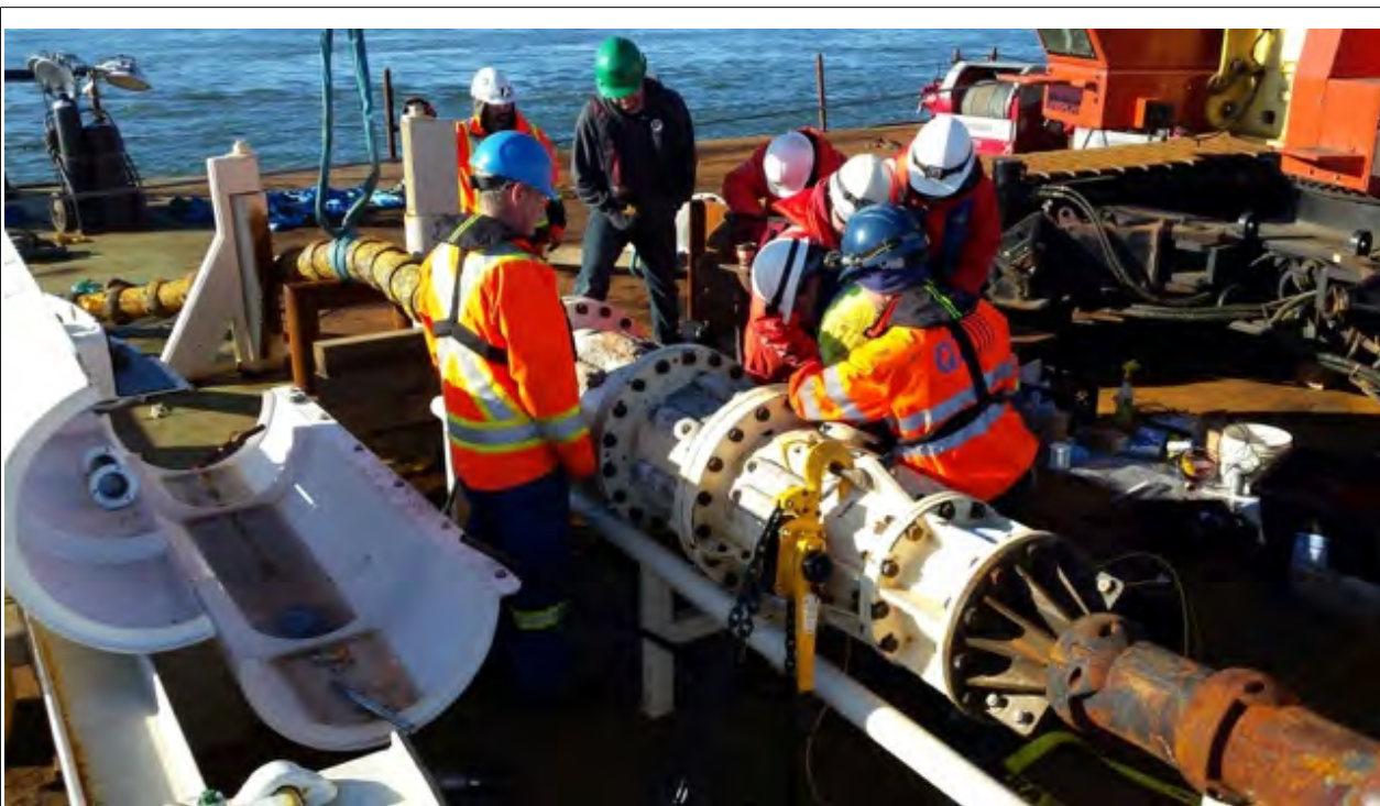
Connecting the cable to transmit power and data to shore.
