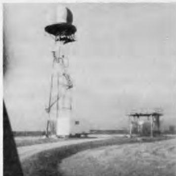
This 50 metre radar tower stands abandoned with an uncertain future. The small platform on the right was the original weather radar installation.
