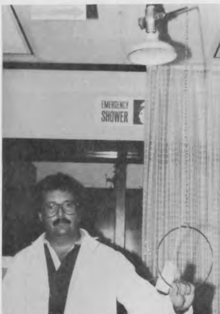
The AES inorganic laboratory is strong on safety features. This emergency shower is located in a central part of the laboratory. Dave Mactavish is just about to pull the chain that would release a shower of water on the laboratory floor. Its main purpose is to counter acid spills. It has yet to be used in an emergency.
