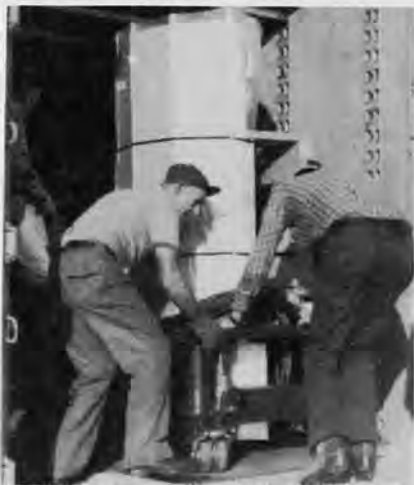
The CRAY computer was delivered by truck to the CMC some four months before inauguration day. Workmen are seen unloading it prior to installation.
