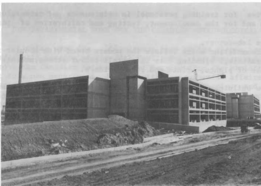
Figure 2. View towards Southeast
