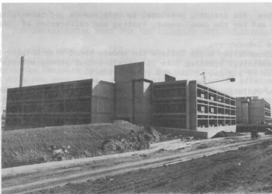
Figure 2. View towards Southeast
