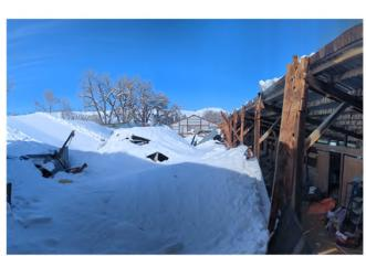
oad, locked in place by a low of -27°F (-33°C), led to this barn collapse on February 18 Photo Credit: Lee Schmelze
